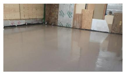
After, outgassed as a result of pouring concrete directly onto aluminium faced insulation
